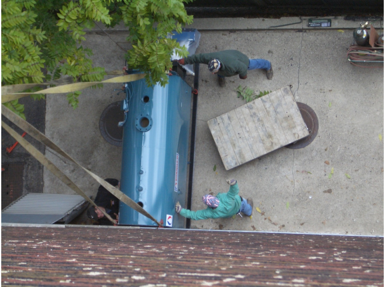
A new boiler gets maneuvered into the boiler room
